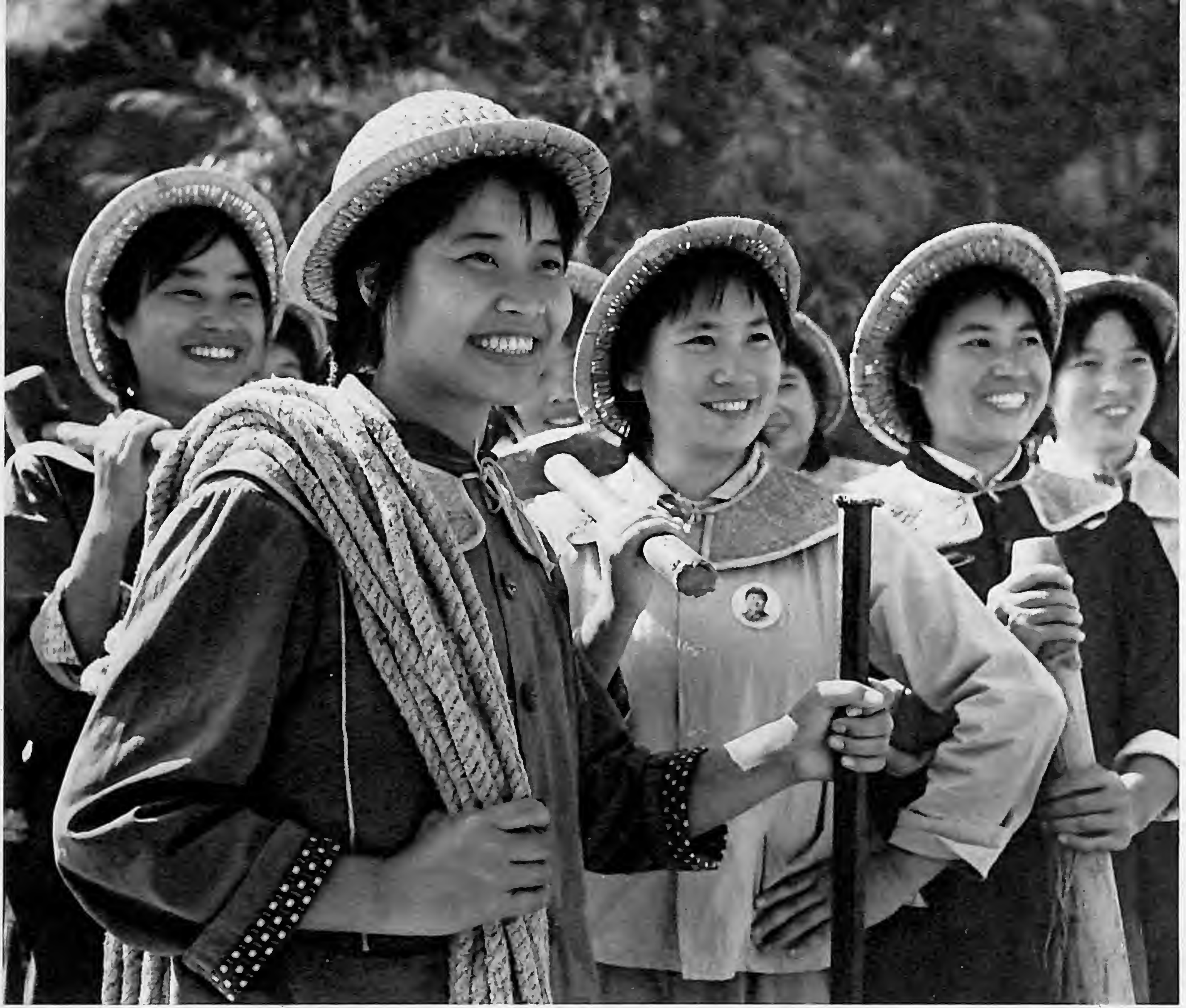
At the Construction Site.
